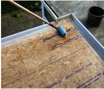
Base resin onto deck
