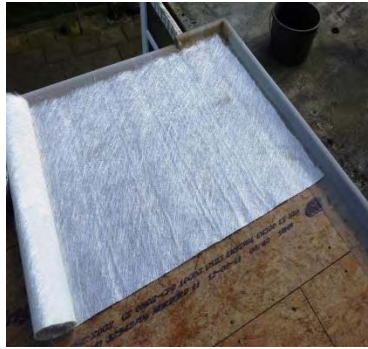
Mat laid into resin
