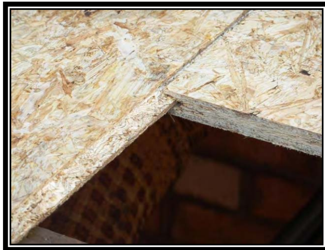
OSB3 tongued and grooved joint
