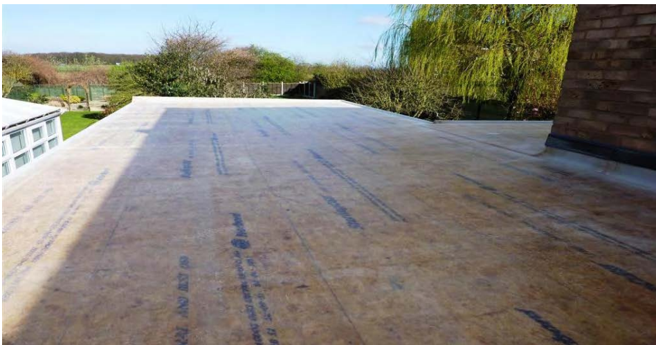
Fully laminated roof – laminate is transparent. Note writing on deck
