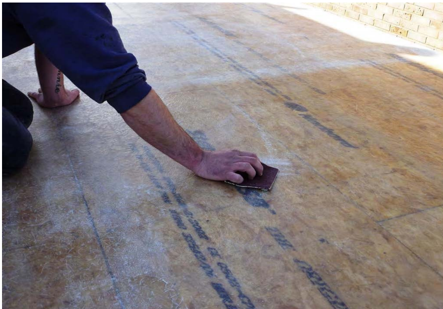
Lightly sanding cured laminate
