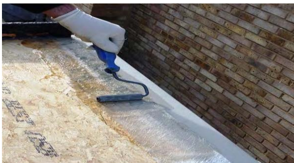
Use paddle to consolidate until transparent
