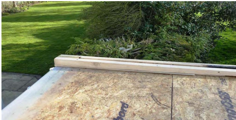
Reverse furring to level front and rear elevations
