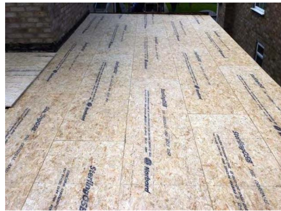
Decking laid – writing facing up
