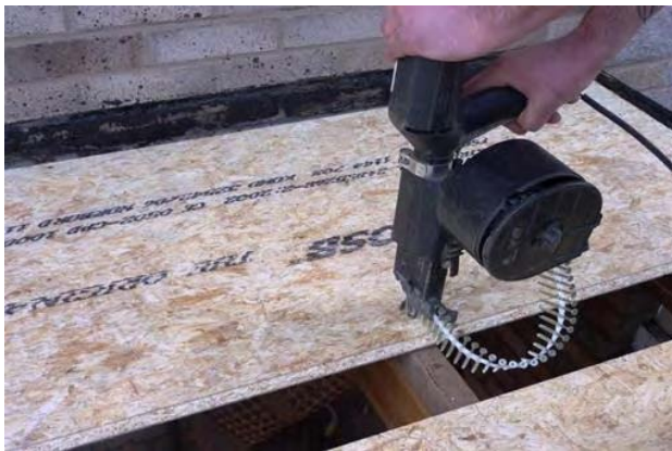
Decking fixed to support joists
