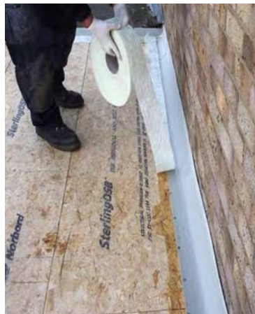
Bandage laid into resin
