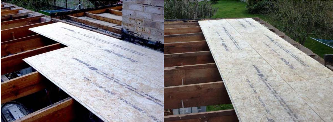
Commence decking (see text)
