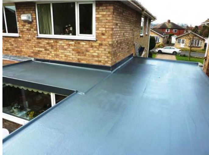
Roof after the TuffStuff® treatment!
