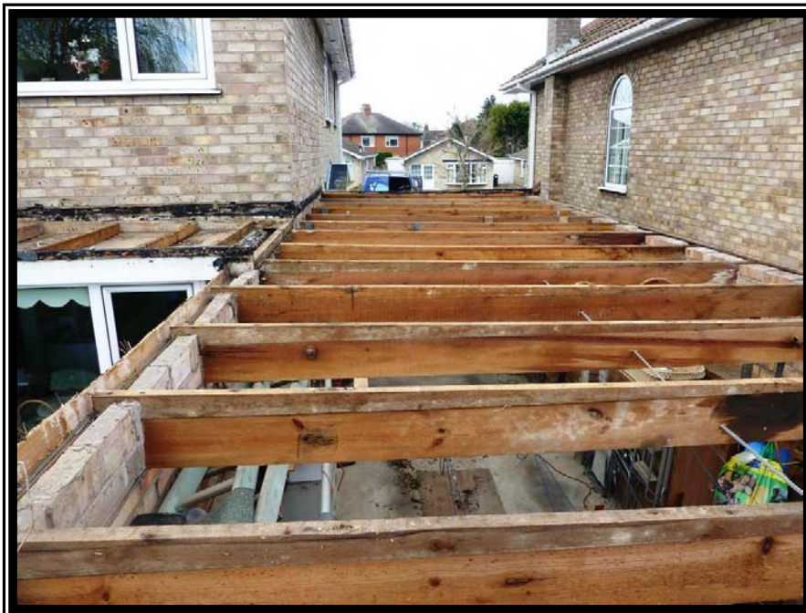
Roof stripped showing firings on top of joists
