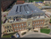
SINGLE PLY ROOFING
