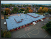
LIQUID APPLIED ROOFING
