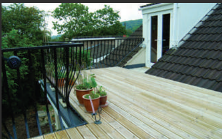
ROOF TERRACES AND BALCONIES
